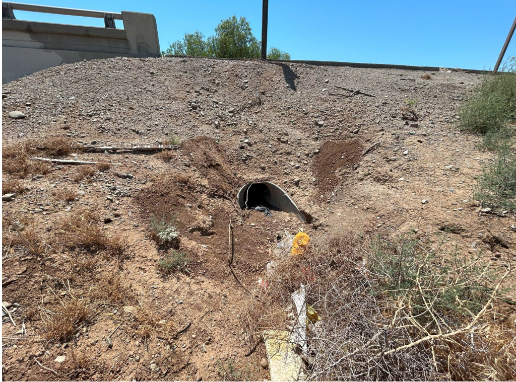
Photograph 5: West corner of Interstate 580/Corral Hollow Road interchange facing south, showing culvert under Corral Hollow Road overpass.
