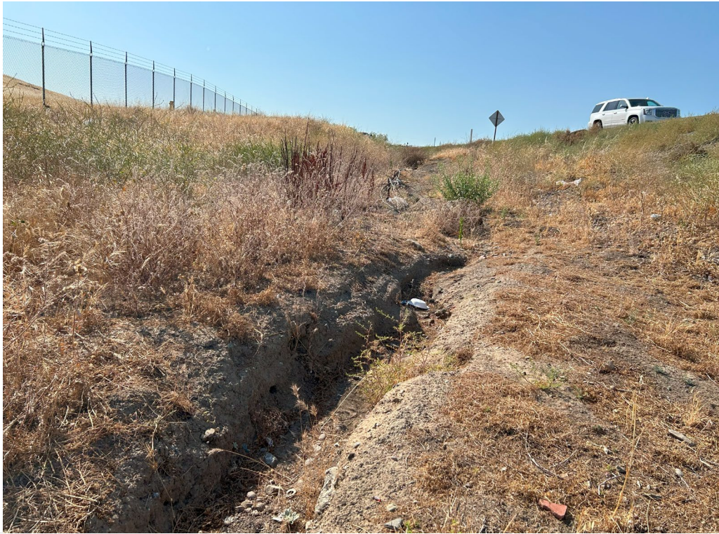
Photograph 9: West side of Interstate 580 in central portion of BSA facing north, showing roadside drainage from cement-lined culvert.
