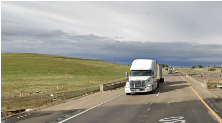
Photograph 3: Northbound view of the I-580/Corral Hollow overpass from the eastbound I-580 lanes near Corral Hollow Creek Bridge. Source: Google Maps Street View.
