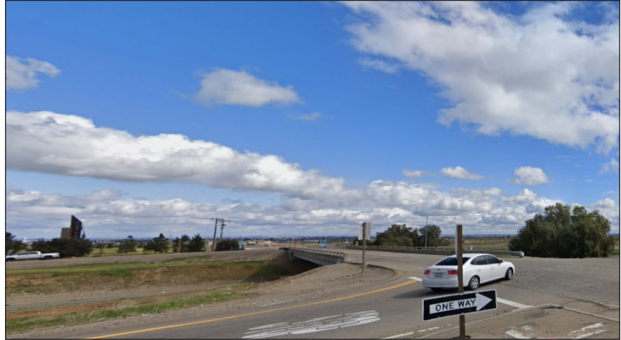
Photograph 2: View of the I-580/Corral Hollow overpass from the eastbound I-580 off-ramp. Source: Google Maps Street View.
