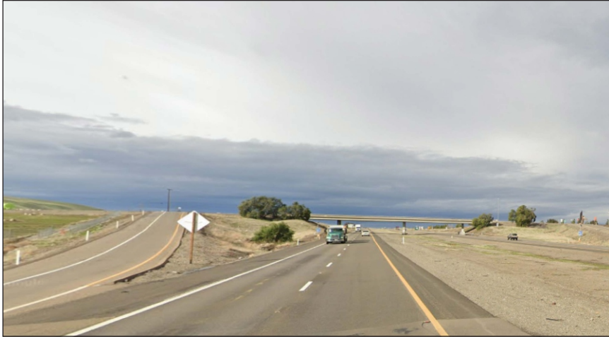
Photograph 1: Northbound view of the I-580/Corral Hollow overpass from the eastbound I-580 on-ramp. Source: Google Maps Street View.
