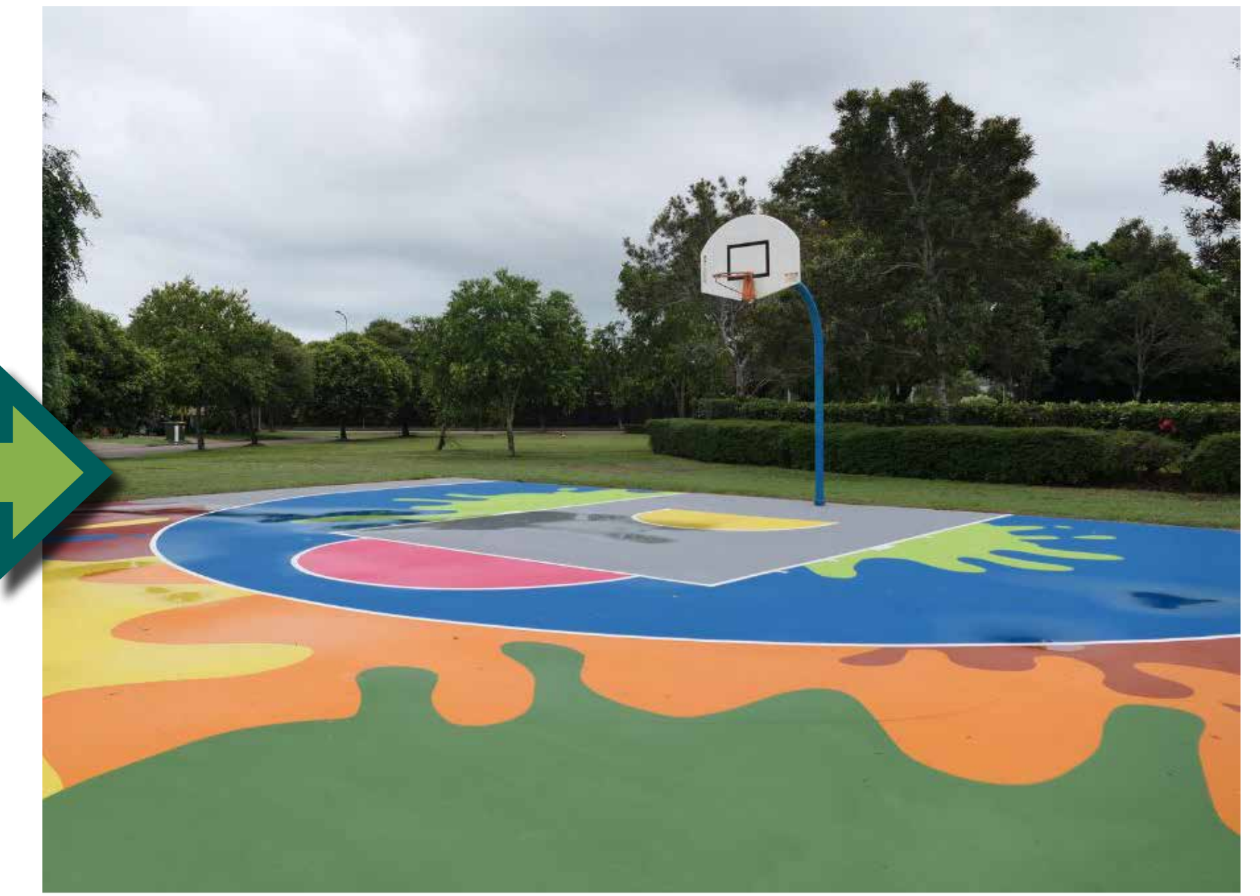
New Court Surfacing
