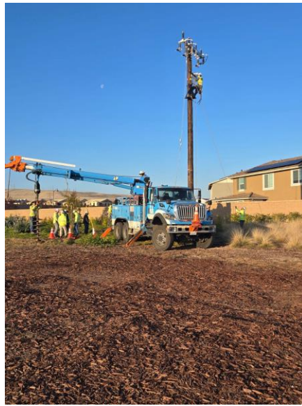
Figure 1. The first electrical pole was installed behind the Parklin community on January 18, 2025. Poles are 80-100 feet tall and approximately 5-10 feet from existing homes.
