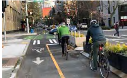
Class IV: Protected Bicycle Lanes/Cycle Track adjacent to the roadway – Source: Seattle Bike Blog
