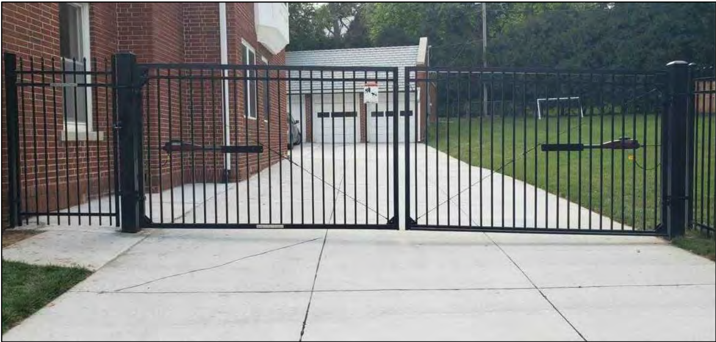
E DOUBLE SWING GATE EXAMPLE NOTE: VEHICLE GATES TO BE 6'-0" MAX HEIGHT.
