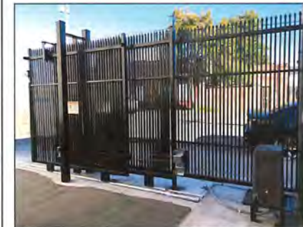
C STACKING/TANDEM GATE EXAMPLE NOTE: VEHICLE GATES TO BE 8'-0" MAX HEIGHT.
