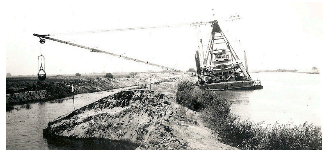
This early 1900s photograph showing dredging work on a levee. (Covello ca. 1900, courtesy of Bank of Stockton Historical Photograph Collection)
