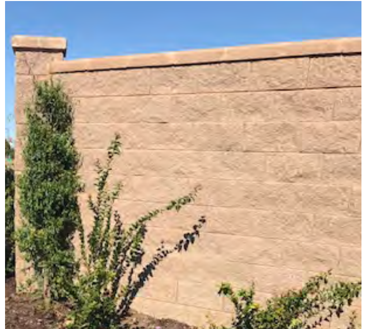
Pilaster: Split Face Column block w/precision cap Wall: Split Face block w/precision cap Color: #113 beigey-brown Basalite product or equal
