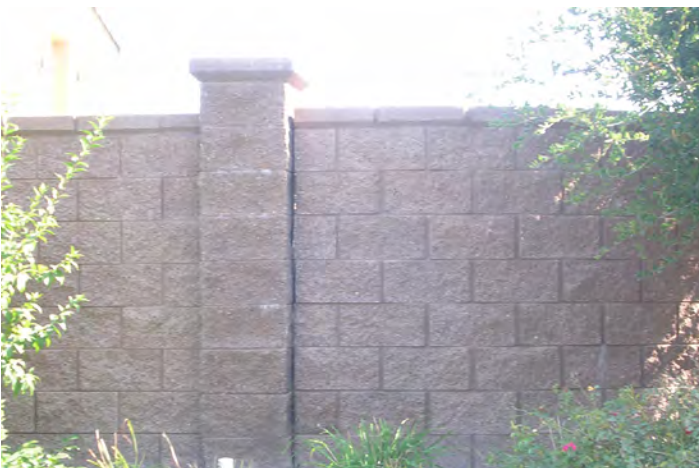
8'-0" Sound barrier/Sound wall acts as a sound barrier, as well as a physical barrier to wildlife, domestic animals and pedestrians.
