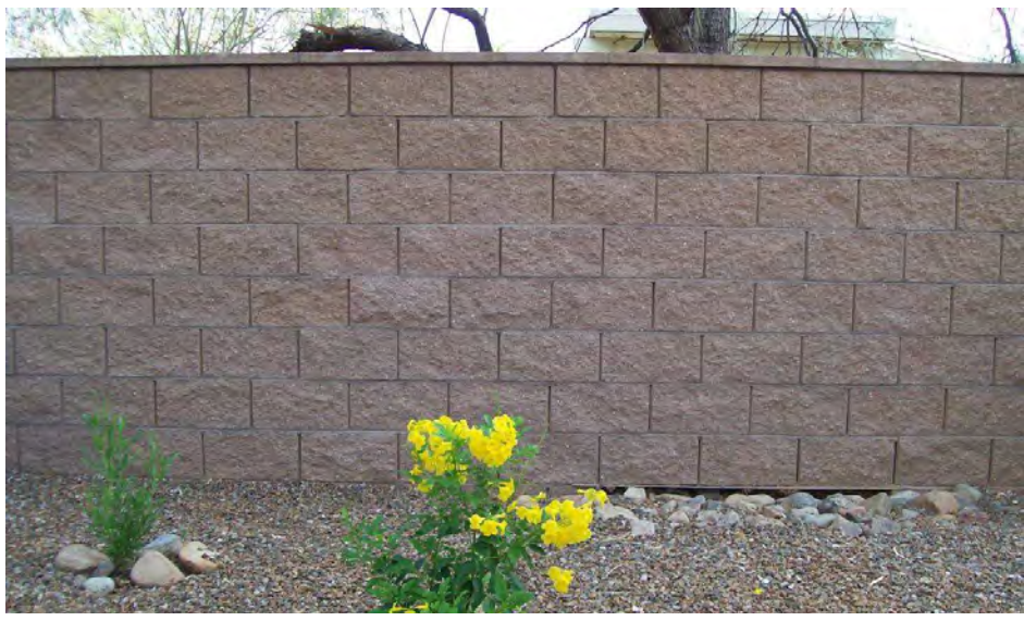
— 6'H Masonry Wall Fence
