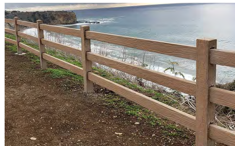
— 42'H Pre-Cast Concrete Split Rail Fence
