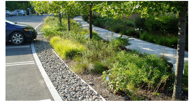
Parking lot with porous surfaces and bioswales
