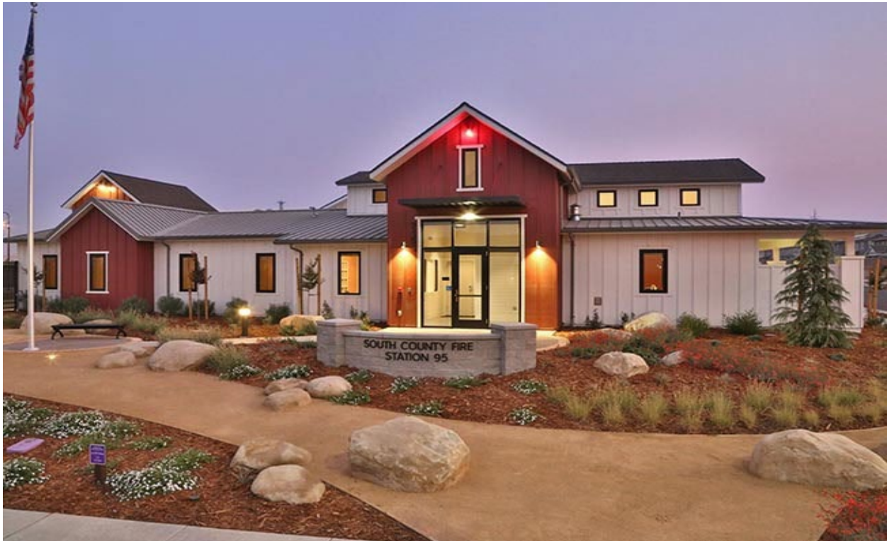
Figure 35 – 2021 Fire Station 95, 7151 Tracy Hills Drive
